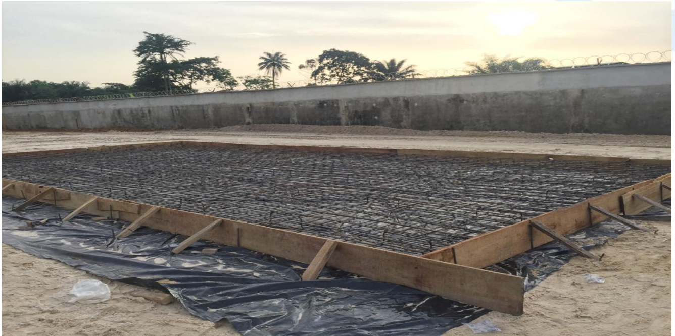
Tab 5.0 – Concrete pouring / Cating
