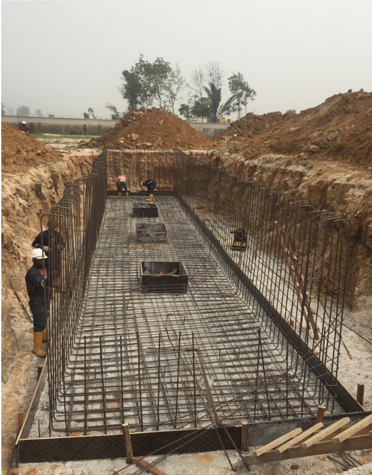
Tab 2.0 – Construction of cellar Pit
