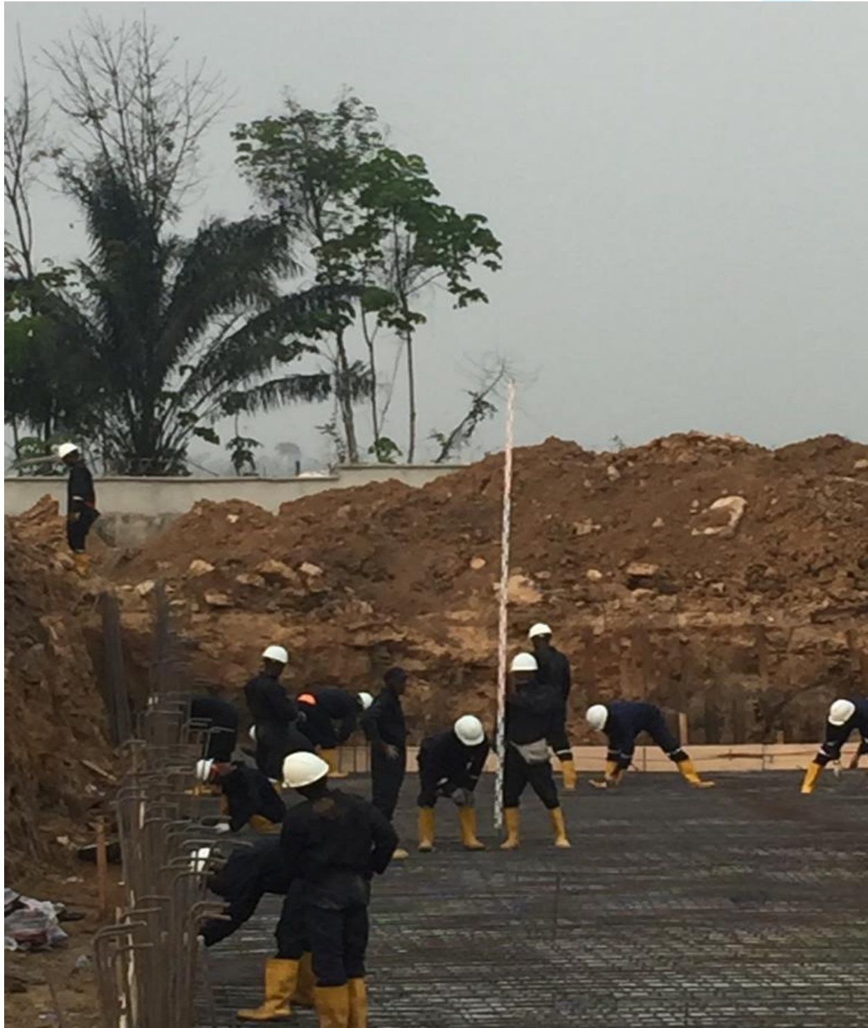
Tab 3.0 – Iron bending in view for concert casting
